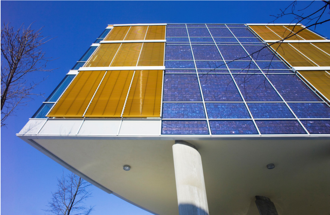
Photovoltaic modules which are integrated into the facade of the building and combined with the SunCarrier reference systems to deliver all the power the competence centre requires.
